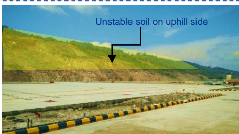
North-west view of the runway
