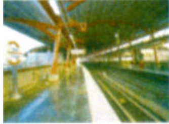
Platform view of Trignagar Metro Station
