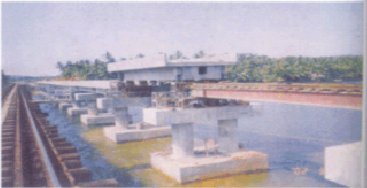
Line Boulding Project Bridge No. 1162 Along Calicut Mangalore
