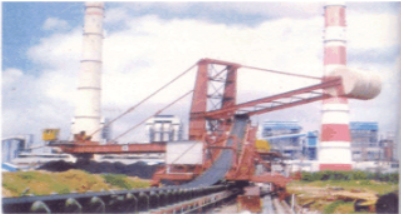
NTPC Talcher Stage-II (4x500MW)- Overall View
